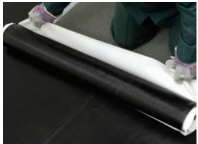
Figure 2 - Application of self-adhesive membranes.
