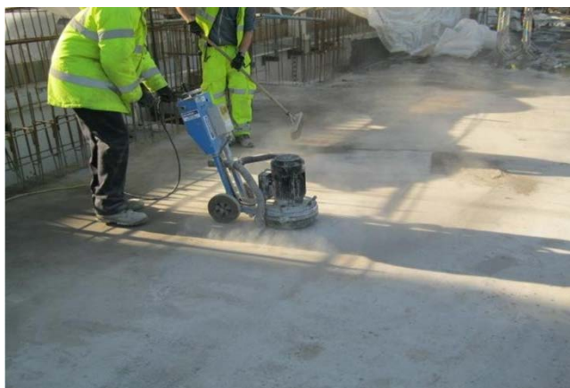
Figure 5 – removal of surface laitance
