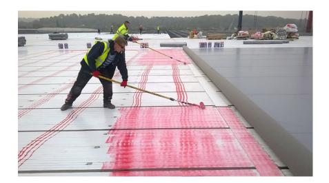
The adhesives can be temporarily placed in a water filled "bitumen boiler" kept at a moderate temperature and monitored; the water should not be heated too high. A suitable risk assessment must be made if adopting such a practice. This however is dependent on each contract allowing the use of a portable gas based system on site.
