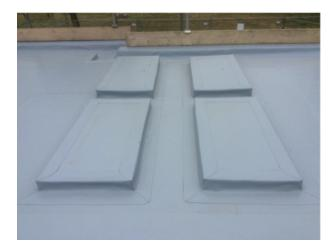
Should a roof area that is fitted with Armourplan PVC or Spectraplan TPE Polymeric membranes suffer from ponding, it will not prove detrimental to the performance or life expectancy of the roofing system, nor will it affect our guarantee.
